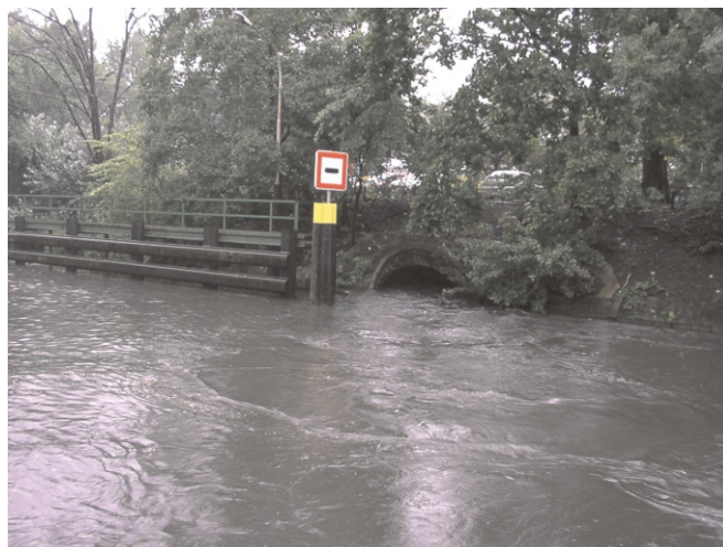
CSO discharge into receiving river
