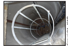
Blick in Brunnen-schacht
