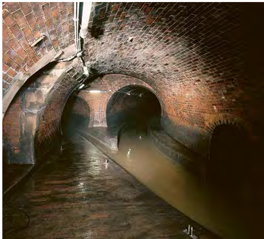
View to a combined sewer system in Berlin
