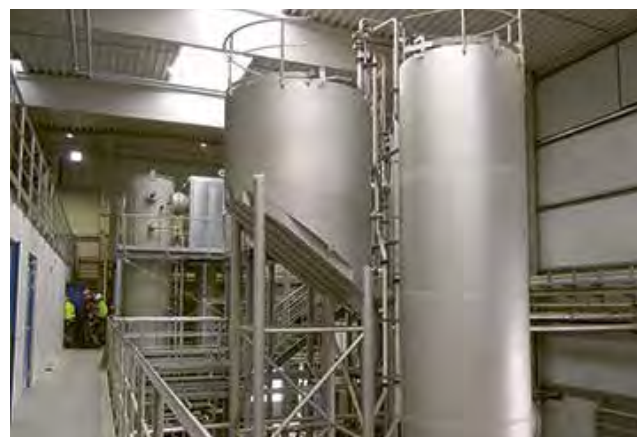
Under construction: plant for nutrient recovery as struvite from sludge liquor (left: precipitation reactor for struvite; right: settler for the sedimentation of the struvite crystals); located at the wastewater treatment plant in Brunswick
