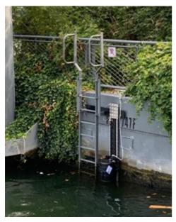
Figure 16: ALERT System V1 installation for long term monitoring in Seine River during DWC campaign
