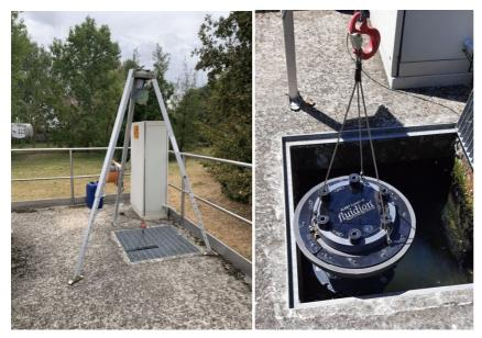
Figure 35: Installation of the Alert V2 at Peschiera Borromeo WWTP
