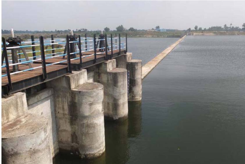
Figure 3: Check dam on Araniyar River in Tamil Nadu (Source: Christoph Sprenger)
