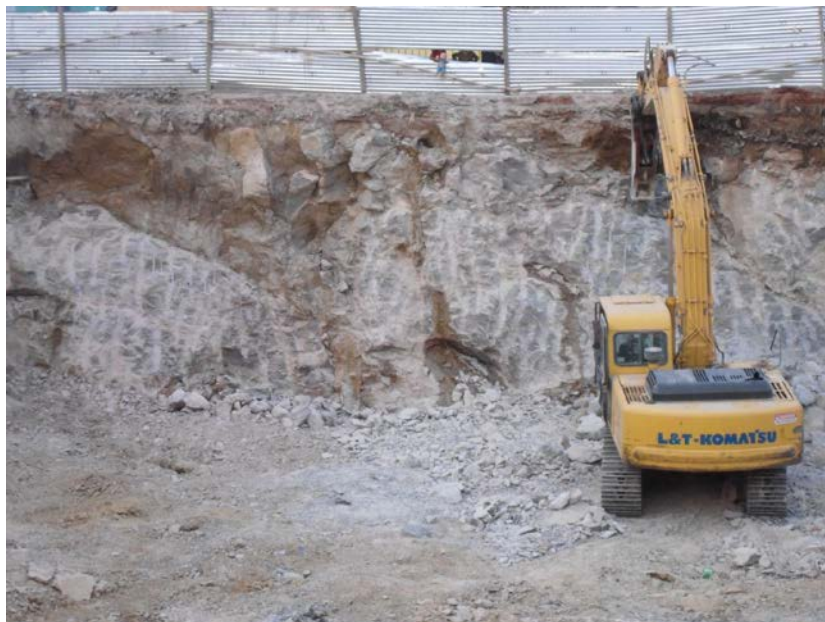
Figure 34. Ongoing construction of recharge structures at a construction site in Raipur.
