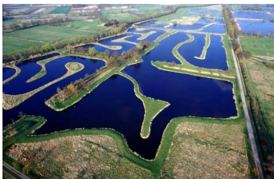
Figure 15: Meander-shaped pond receiving effluent of WWTP Brunswick (from Abwasserverband_Braunschweig 2008).
