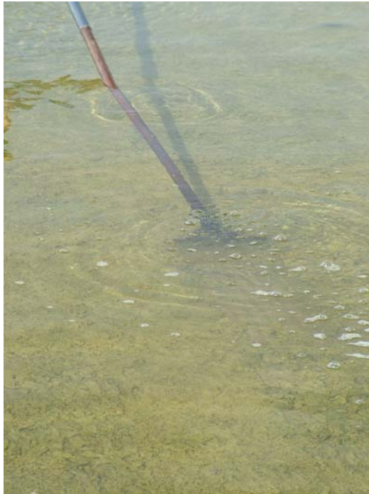
Figure 40: Photograph taken during raking of the SSF in order to destroy the superficial clogging layer.
