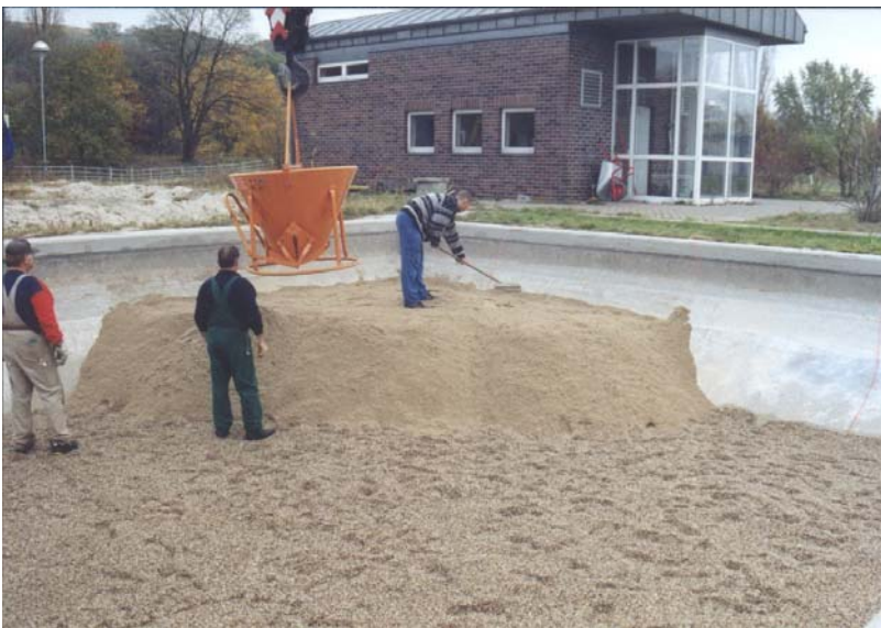
Figure 37: Preparation of the filter sand during sand exchange.
