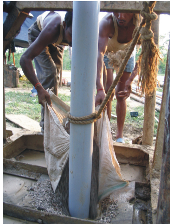
Foto 4 Backfilling with pea gravel
