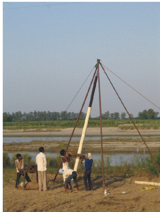
Photo 2 Rig for manual drilling and assemblage.
