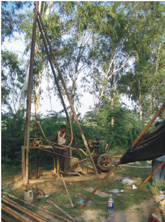
Foto 3 Rig for rotary drilling
