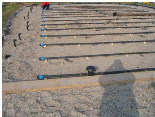
Fig. 2.4.18: Constructed wetland, distribution system
