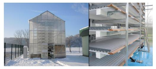
Figure 6 Left: Front view of Greenhouse containing the APS duckweed plant; Right: duckweed plant trays of the APS system inside the greenhouse
